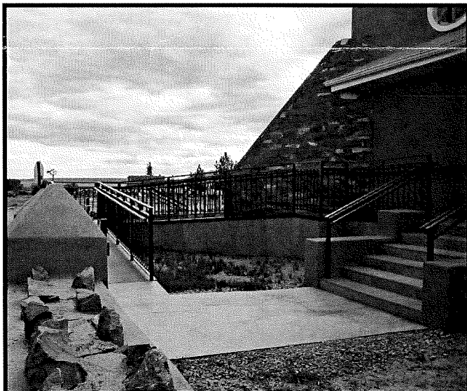
New Handicap Ramp at the Church (See story, p.2)
